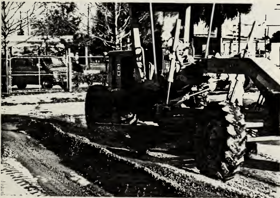
Figure 2.16 Grader Windrowing Wet Material
